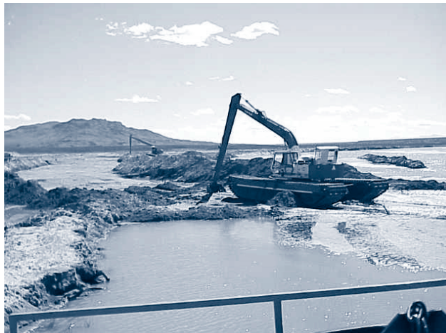
ISC Amphibious dredge for excavating the Elephant Butte pilot channel.
