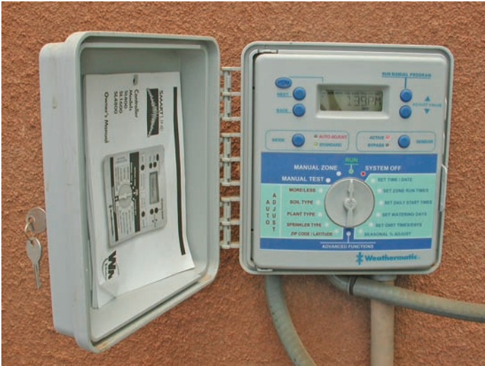
Figure 10-6: An irrigation controller can be programmed to automatically turn each zone of your irrigation system on and off.
