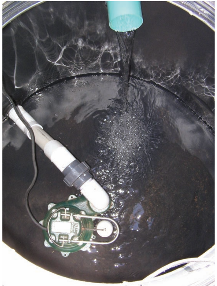
Figure 10-1: A sump pump must be submerged in water in order to work.
