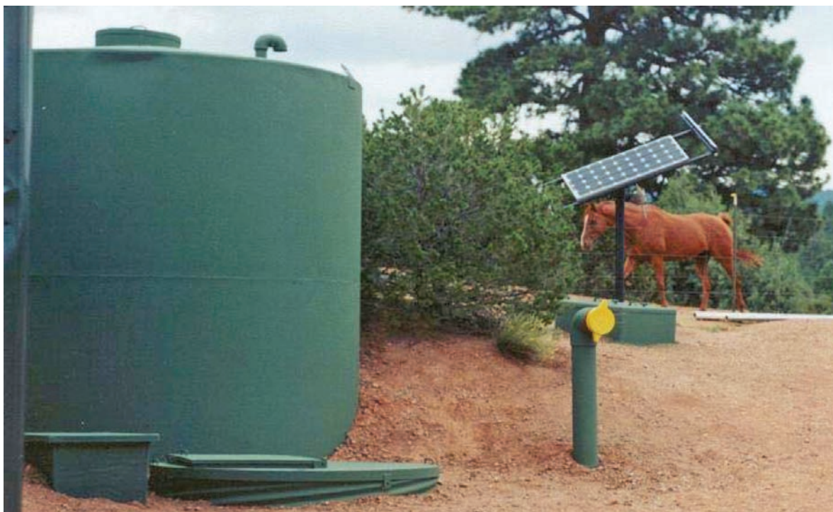
Figure 2-3: An example of an aboveground cistern system storage tank with a solar-powered pump.
