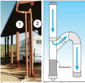
Figure 8-11. Roof water is initially conveyed from the downspout into a pipe (#1) that dead-ends (preferably near a planting bed). After that pipe fills, the cleaner water flows through pipe #2 to a cistern. The cutaway illustration shows how sediment settles in the first pipe.
