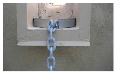
Figure 8-7: A rain chain is a simple but effective way to direct water downward from a canale.
