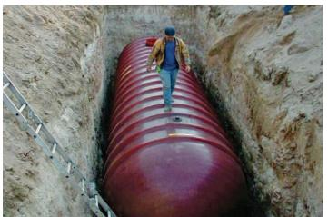
Figure 9-9: A fiberglass tank being installed.
