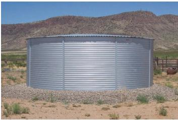
Figure 9-10: Steel tanks are a cost effective option at 5,000 gallons and larger.
